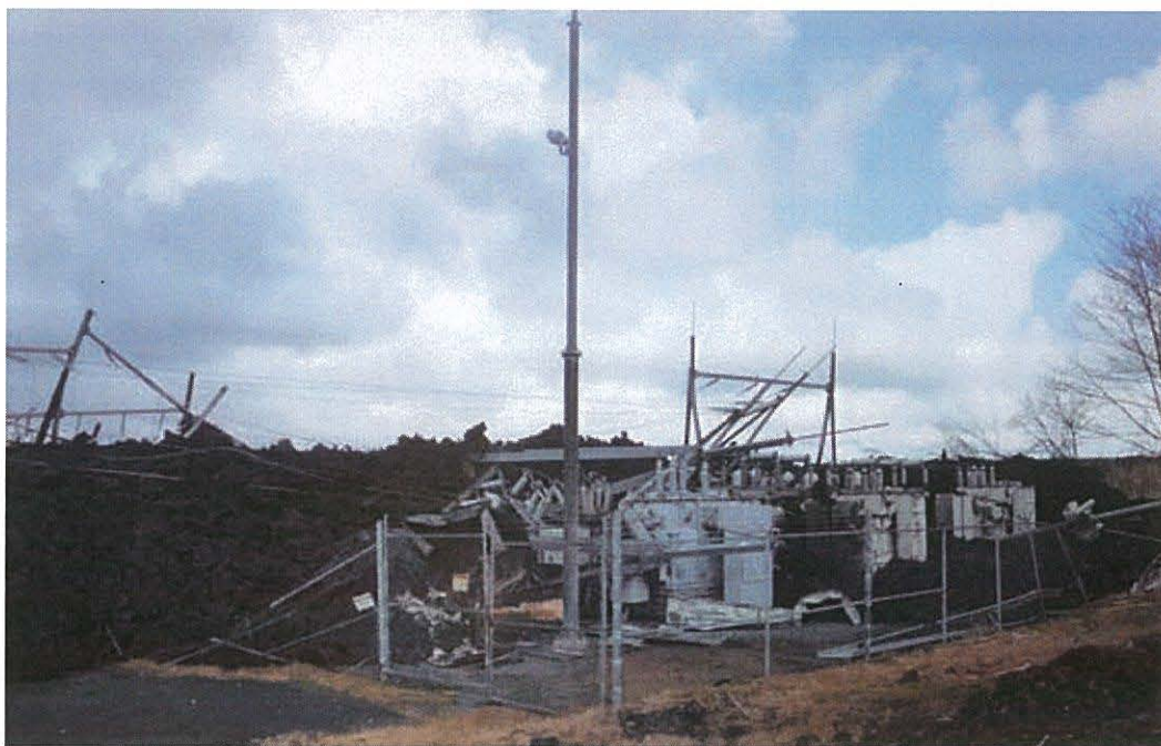
Figure 2 - Pictures of overrun switching station (looking from PGV plant side)
